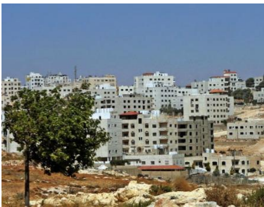
Figure (3) the different in building height in one area.
