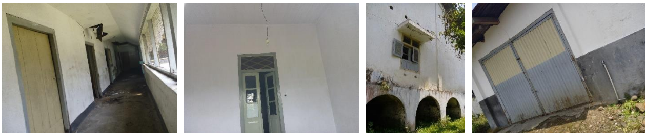
Figure 6. Door and window shape of first house.
