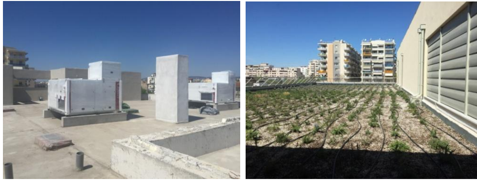
Figure 11. a) Wind chimneys on the roof; b) green roof
