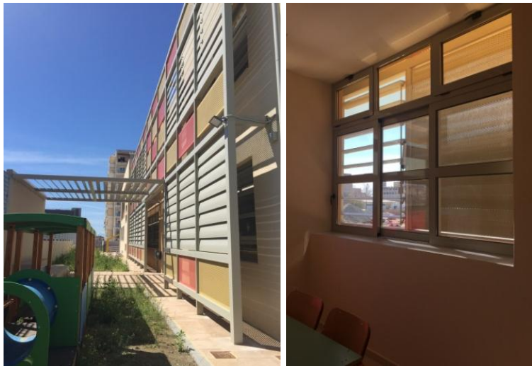
Figure 9. a) Exterior shading blinds; b) shading enhancement of the classroom
