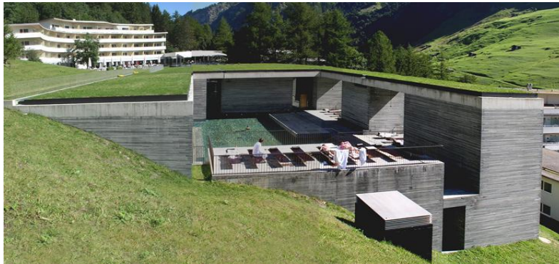
Figure 9. Thermal Vals, Switzerland
