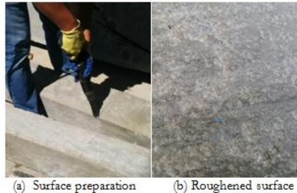
**Fig.5. Surface preparation and roughened surface**
