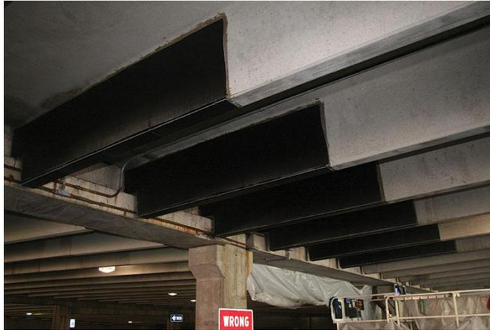
**Fig. 1. CFRP strengthened concrete beams**
