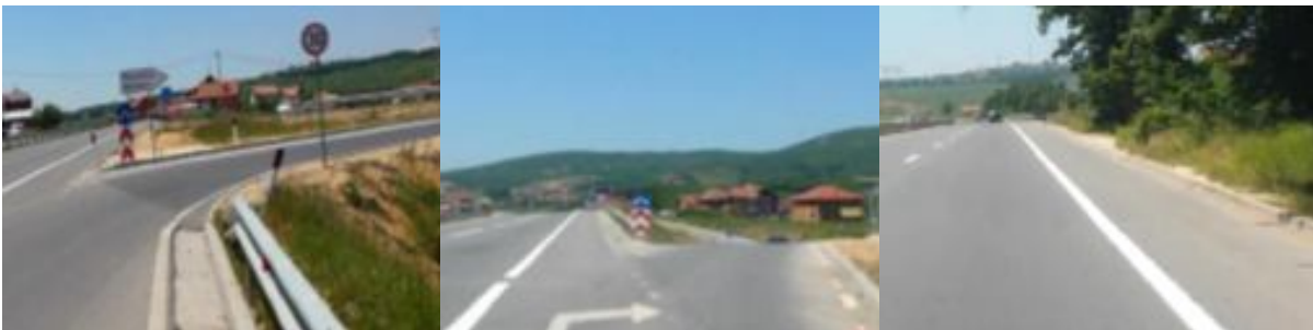
a) Low circular radius b) Low vertical radius, c) Narrow emergency line
