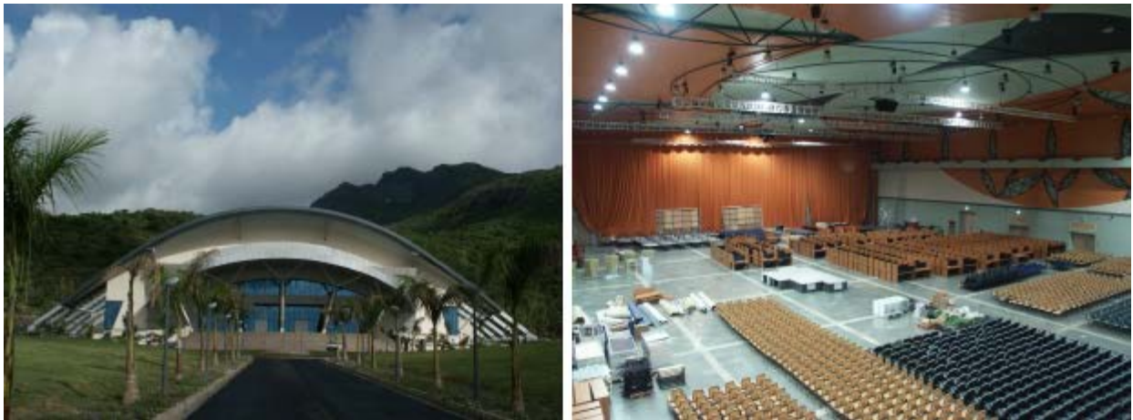
Fig 1: External and internal view of the polyvalent hall
