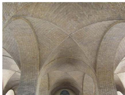
**Fig. 5: Arg Square in Kerman. Master Builders Built Groin using an arc that goes Through Three Points (Photograph by the Author)**
