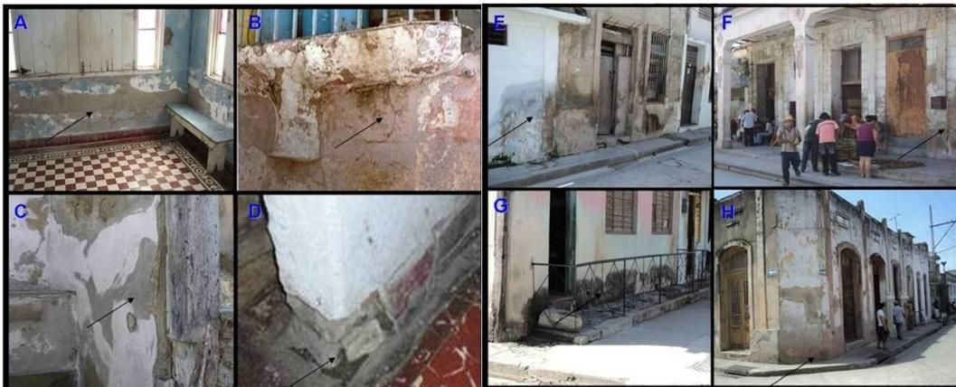
**Figura 3: Attack of the Capillarity Humidity in Buildings of the Study Area. A, C y D: Inside Houses Locations; B, E, F, G y H: Facades**
